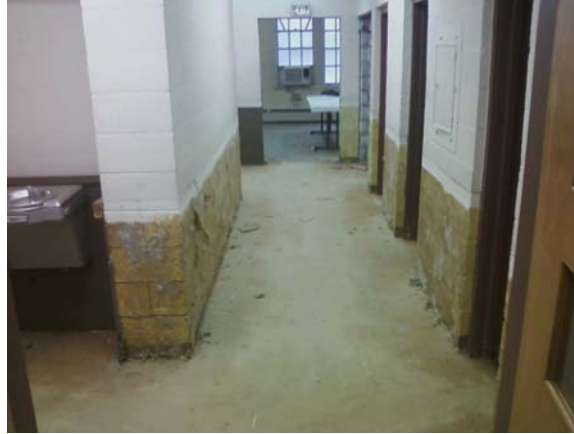
Hall way going from Fellowship Hall to Lounge area
