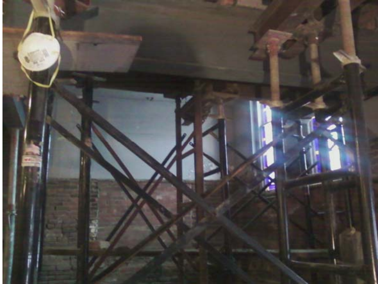
Beam in Fellowship Hall
