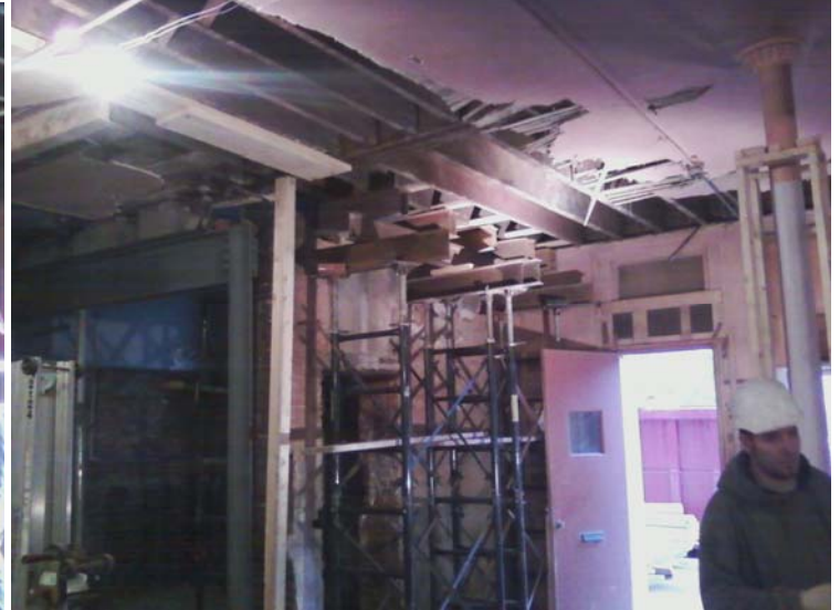
The first steel beam in Fellowship Hall is now in place. The second wall will be removed on Tuesday
