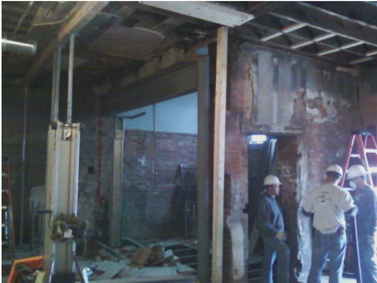
The first steel beam in Fellowship Hall is now in place. The second wall will be removed on Tuesday
