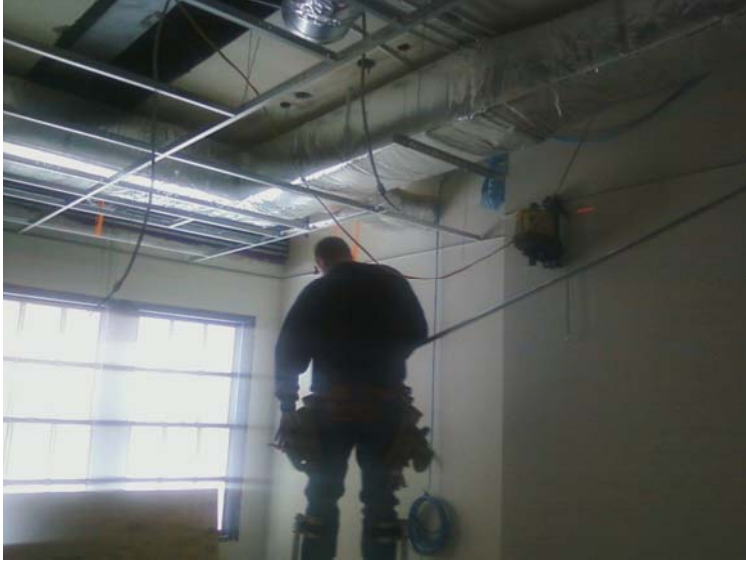
Pictures show the ceiling grid being attached in the offices.
