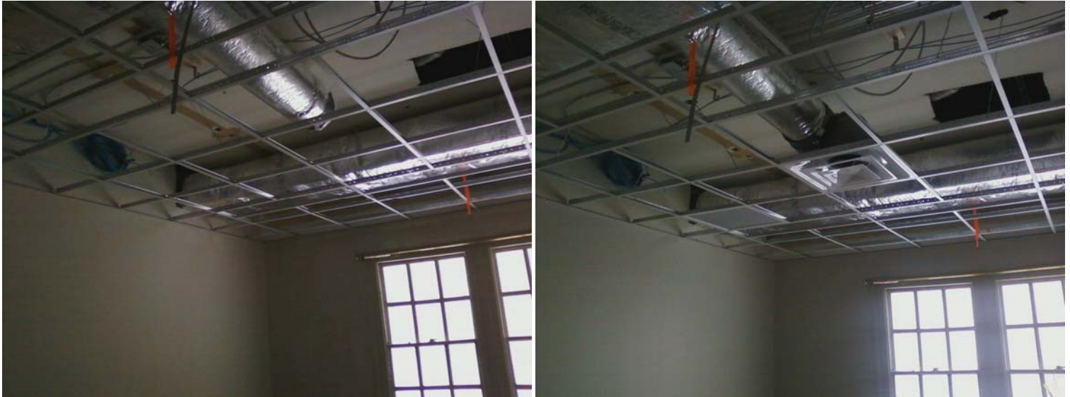
Dust work and ceiling grid along with the new HVAC deflectors.
