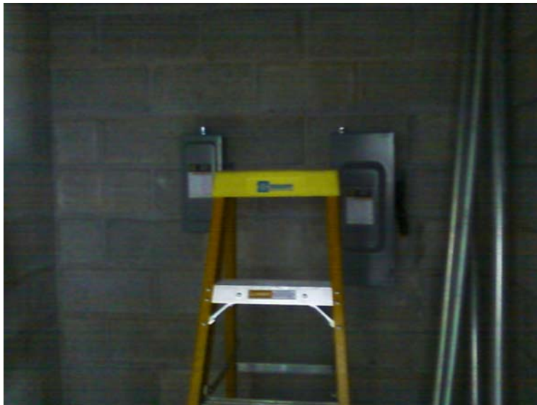
Electrical boxes being installed in the elevator lift room.
