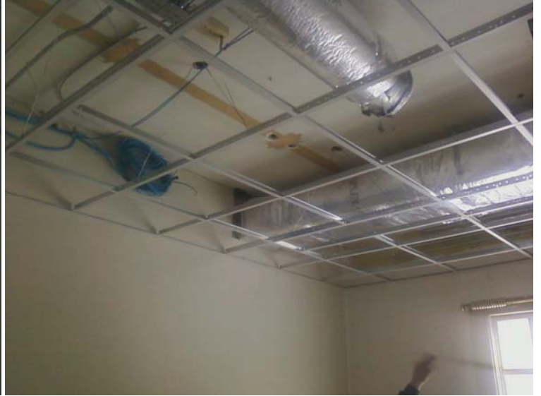
Pictures show the ceiling grid being attached in the offices.
