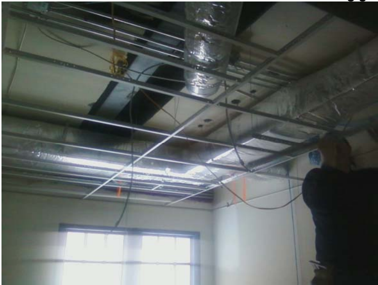
Pictures show the ceiling grid being attached in the offices.
