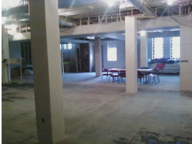
Picture of Fellowship Hall with applied drywall ready for joint compound and tape to be applied.
