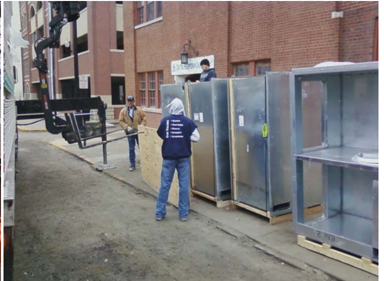
Drywall truck unloading and HVAC group preparing the curbs to be located to the roof.
