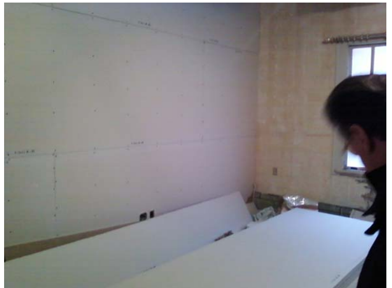
Drywall installation in Pastor's and Asst. Pastors office
