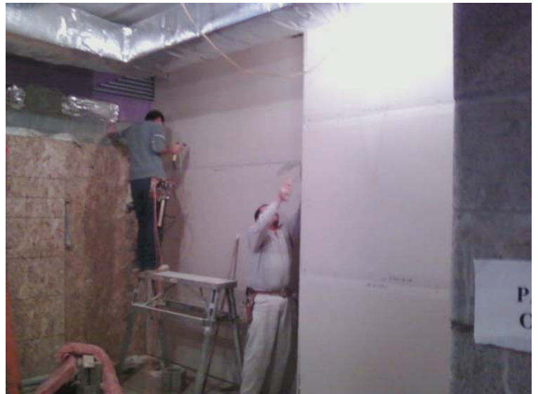
The drywall baffles in Sarah's new office and the drywall going up in Lant's new office area.
