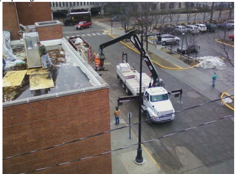
Pictures show the curbs being lifted to the roof in anticipation of the five new heating/air conditioning units that should arrive in March.
