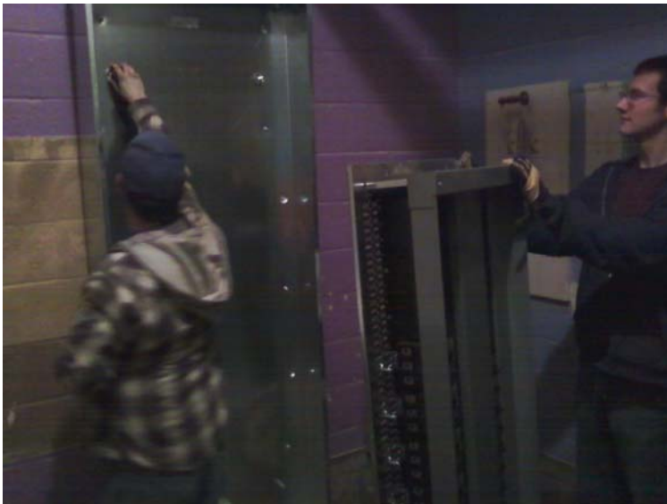
The breaker panels are being delivered for the electrical room and the preparation for the new entry an electrical service is being prepared. The last picture shows the northeast corner of Fellowship Hall with drywall. Notice the enclosed track for the movable walls.
