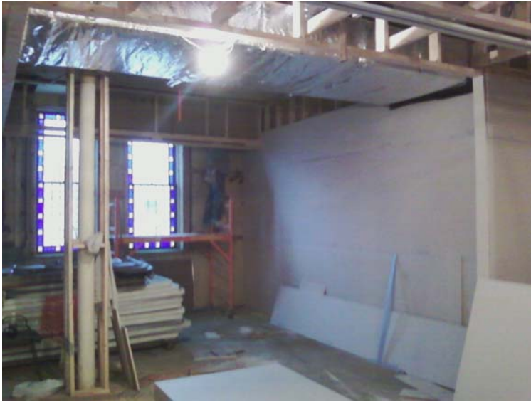
Picture shows the drywall going up in Fellowship Hall and the HVAC group working with drywall installers to finish the Fellowship Hall installation.
