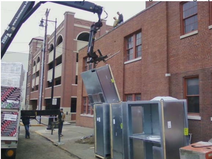
Pictures show the curbs being lifted to the roof in anticipation of the five new heating/air conditioning units that should arrive in March.
