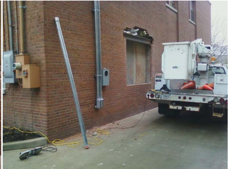
The masons are installing the new window in the Pastor's office and the outside electrical entrance equipment is being prepared. Thursday – January 21, 2010
