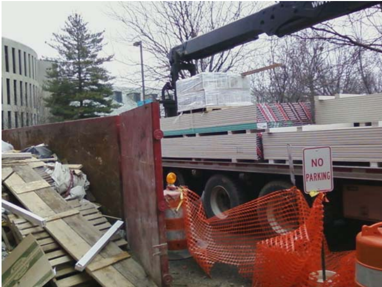
Drywall truck unloading and HVAC group preparing the curbs to be located to the roof.
